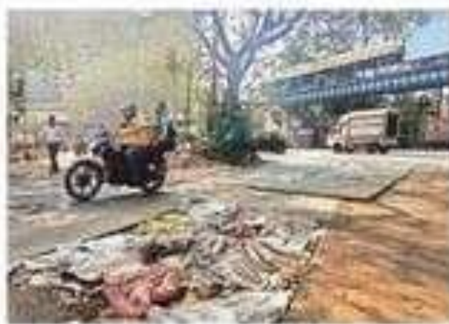
A large pothole near the junction of Barmer Nath Path Road and Cotton Green railway station. The pothole, reportedly caused by recent road work in the area, has been temporarily patched with sacks. Anil Chatterjee
